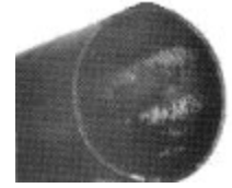
Pipe after PKU device
